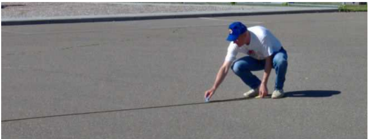
Preparing to stripe the parking lot
